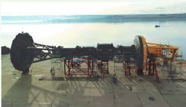
PB150 at dockside awaiting deployment in Scotland
