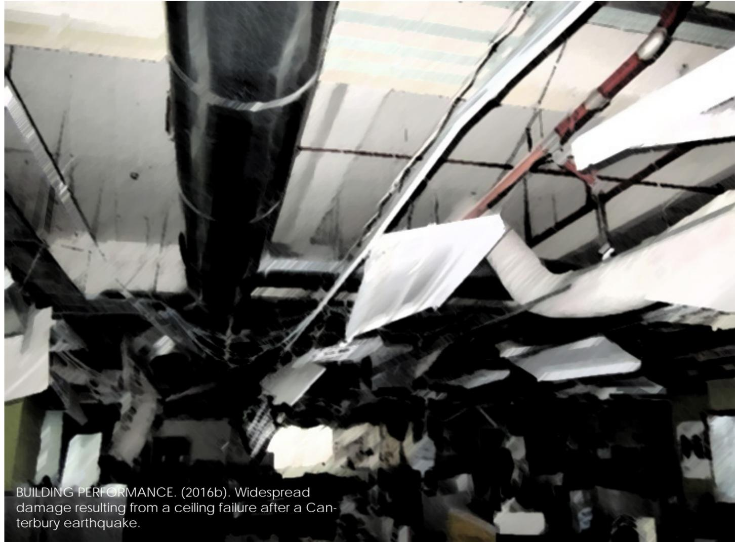
BUILDING PERFORMANCE. (2016b). Widespread damage resulting from a ceiling failure after a Canterbury earthquake.
