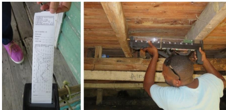
Figure 6. Using the resistograph in a rafter under the floor (Flores, 2018)
